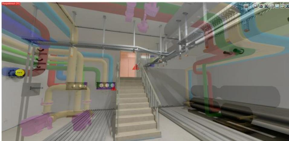
FRAMENCE: BIM-Modell (as planned) versus Realität (as built)
